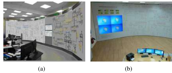
Figure 2. Examples of visual management information centers: (a) complex solution of the company POISK [7]: mnemonic scheme, plastic appliqué, LCD panels; (b) S - 2000 dispatch board, built-in video cubes of NTK Interface LLC [8]
